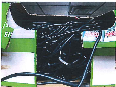
Box of power cables (15)
